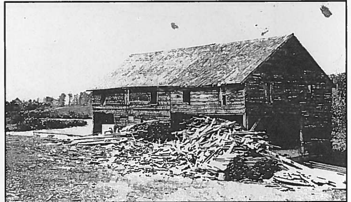
A historic photograph of the wooden-framed Chick's Mill and lumber yard. The mill pond is to the left. Logs stored in the pond were drawn up a ramp on the left end. Sawn lumber was removed on the right end, and waste was tossed through the opening on the side.
