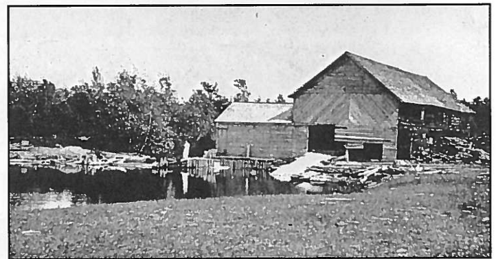
A second historic photograph view of Chick's Mill from the mill-pond side. The dam is to the left of the ell that rests on it. (Both of the historic mill photographs are after Wakefield-Brookfield Historical Society 2006:90.)
